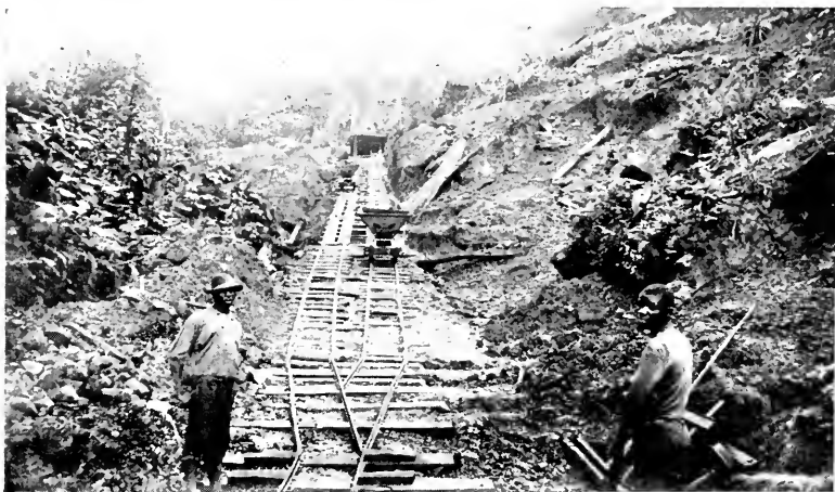
A GRAVITY INCLINE, THE LOADED CAR PULLING UP THE EMPTY ONE.
